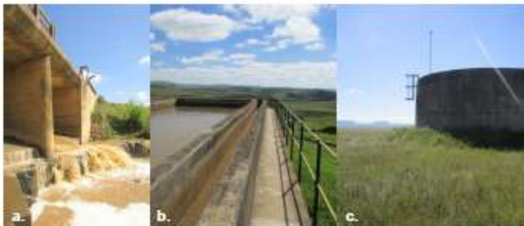
Figure 1: The existing LRWSS which transfers water from a weir on the Xura River (a) to the water treatment works (b) and then storage reservoirs (c).
