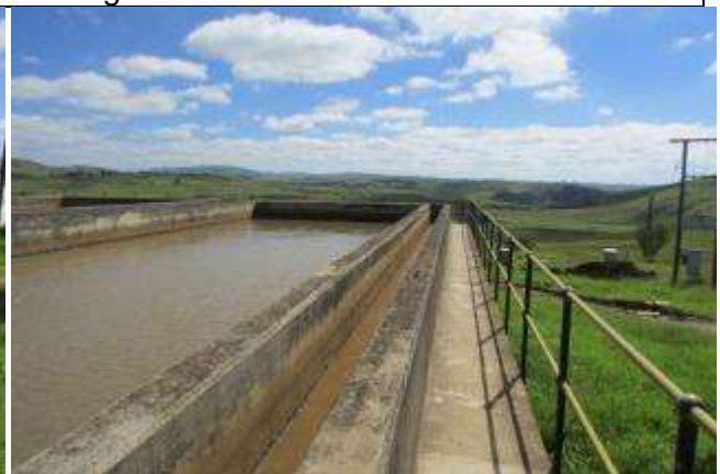
The deflocculation ponds at the existing water treatment works.
